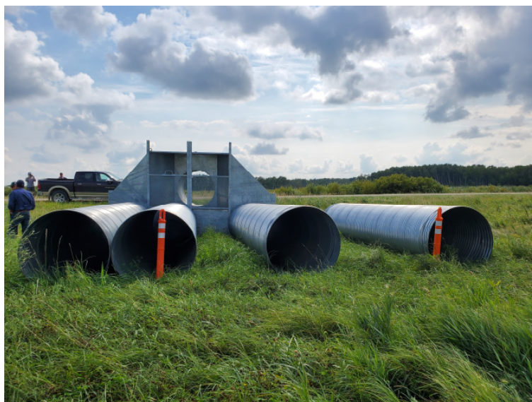
Culverts ready for installation at DeBlonde Water Retention Project
