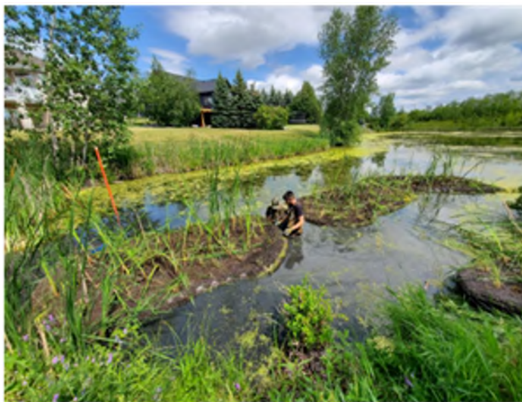
Floating treatment wetlands in stormwater retention pond in East St. Paul, MB.
