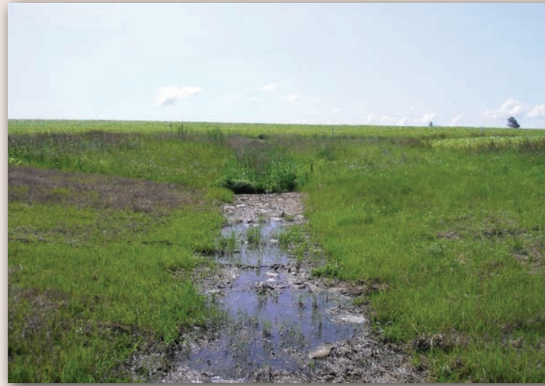
Surface runoff control measures such as rock-lined waterways (above) and buffer strips, were found to improve water quality in the Fourchette Watershed.
