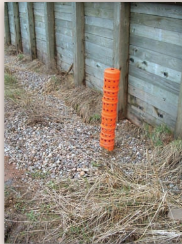
The storm water diversion BMP was installed to collect storm water from barn roofs and divert it past manure handling areas, in order to reduce the contamination of surface runoff en-route to the stream.
