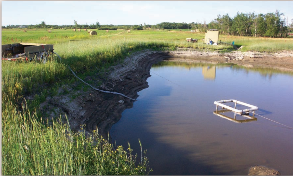
The small holding pond downstream of the winter cattle containment area was found to reduce nutrients and E. coli loadings to the stream but the construction of the pond requires a high capital investment.
