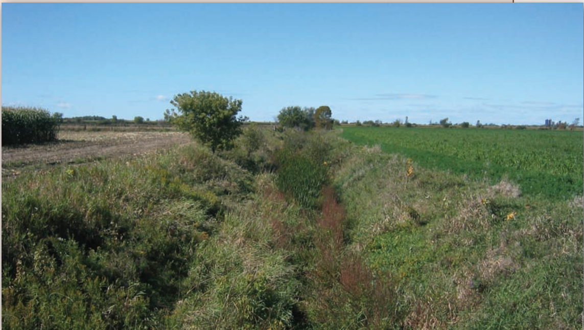
The tile drainage underlying much of the WEBs project site in the South Nation Watershed empties into a series of ditches and municipal surface drains.
