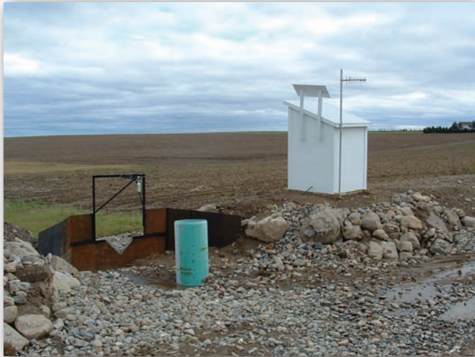
Automatic sampling stations help keep track of periodic runoff events.
