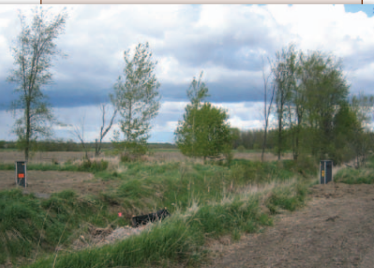
Controlled tile drainage structures have provided clear economic returns to the producer.
