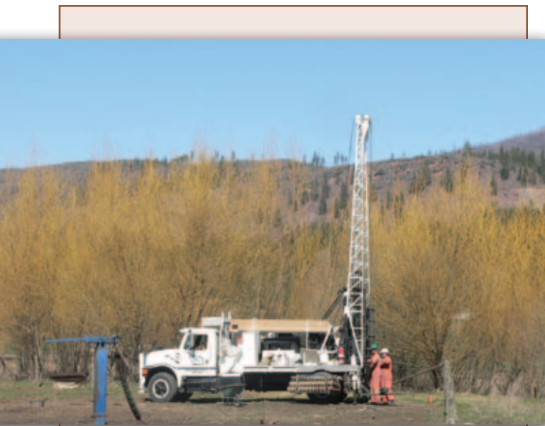
Small-diameter wells were installed in the Salmon River Watershed to monitor groundwater quality.
