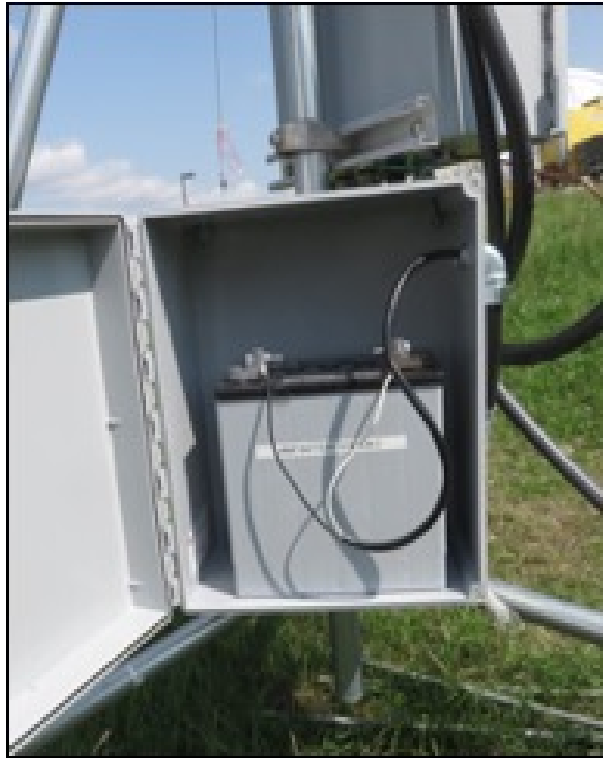
Figure 2.5: External 12V battery inside battery housing box.
