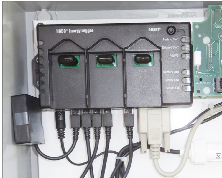
Figure 3.1: Completed SmartSensor Set-up.
