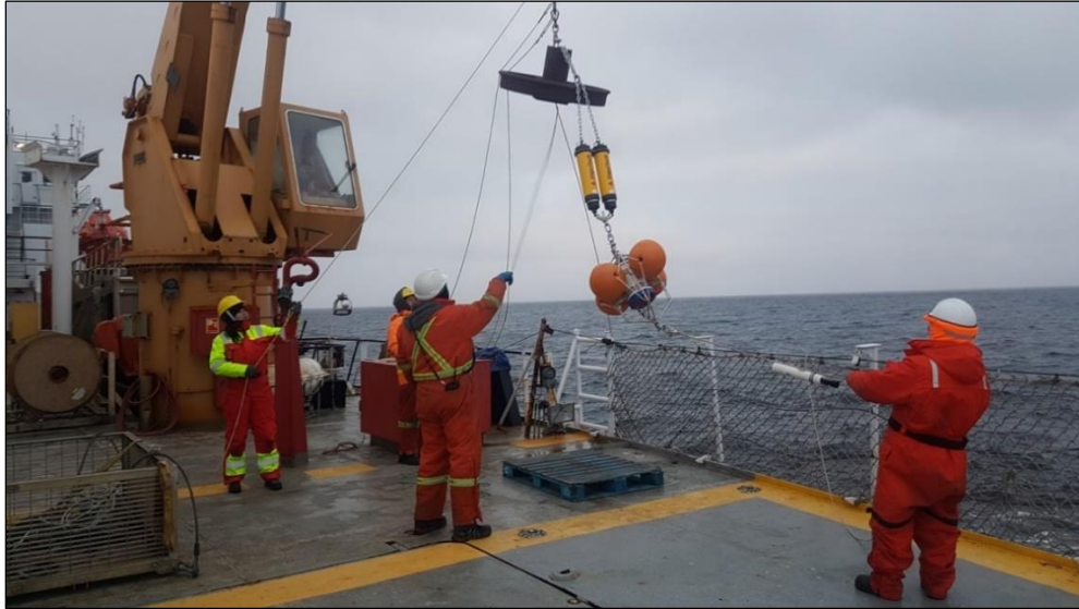
FIGURE 6.5 Mooring deployment from the helicopter deck
