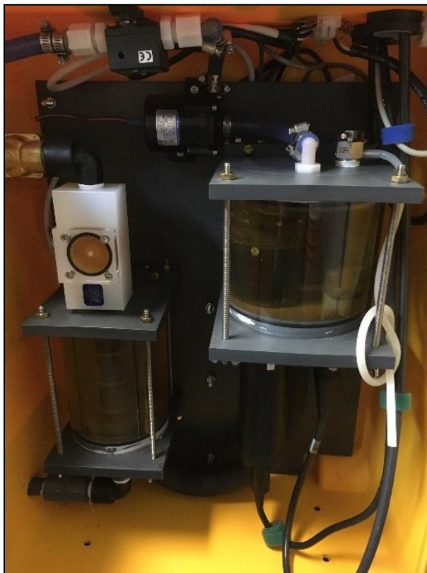
FIGURE 7.35 The underway optode / GTD (PIGI) system installed in the forward lab
