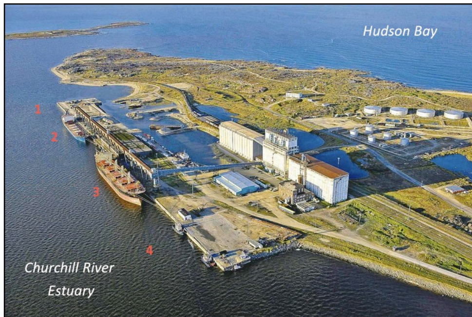
Figure 3.1: The Port of Churchill’s wharf and shipping berths ( Port of Churchill , n.d.). Photo modified from Winnipeg Free Press (2013).
