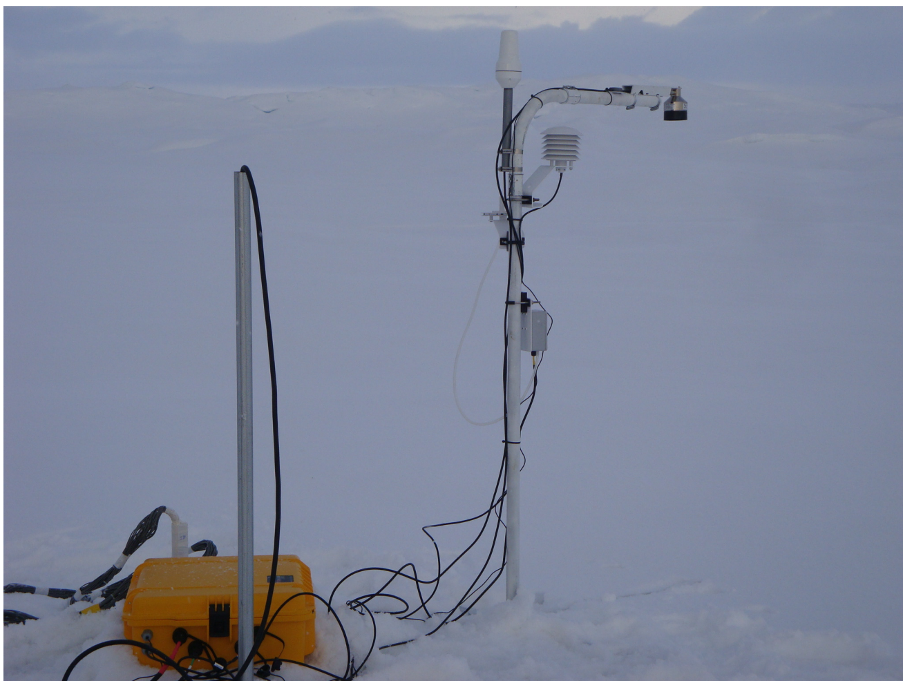
Figure 20: CEOS IMB04 installed on 27 September 27 2010 in the Beaufort Sea.
