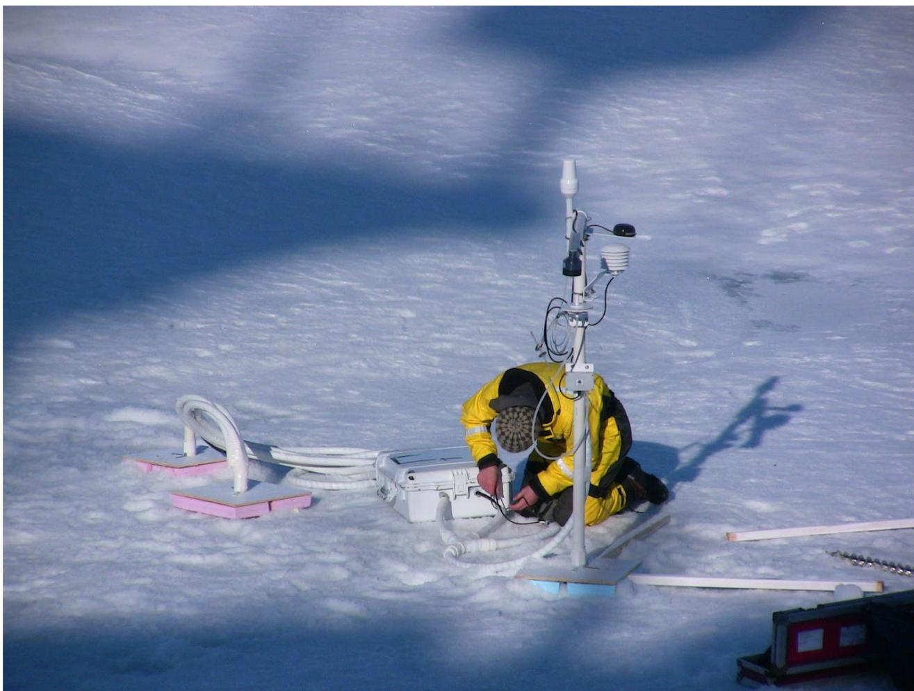
**Figure 43:** Ice Mass Balance Buoy Installation by 09 September 2009 at station L1.1.
